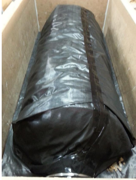
Figure 4 SK75 Test Unit Installed in the Test Tank Prior to Backfilling
