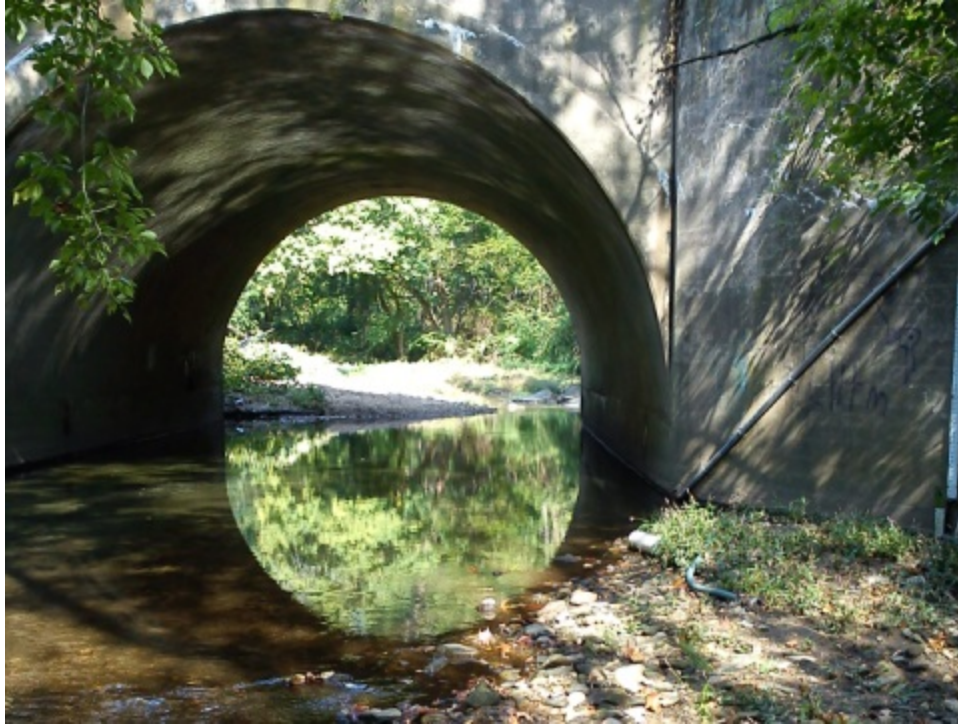
Figure 23. Gage 01475530, Cobbs Creek at Rte. 1, looking upstream
