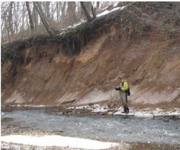
Figure 1. Eroded stream bank at Poquessing Creek times when the public is most likely to be near or in contact with the stream. In dry weather, stream water quality should be similar to background
