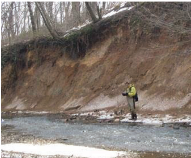
Figure 1. Eroded stream bank at Poquessing Creek
