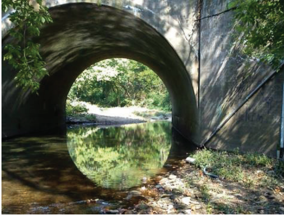
Figure 23. Gage 01475530, Cobbs Creek at Rte. 1, looking upstream
