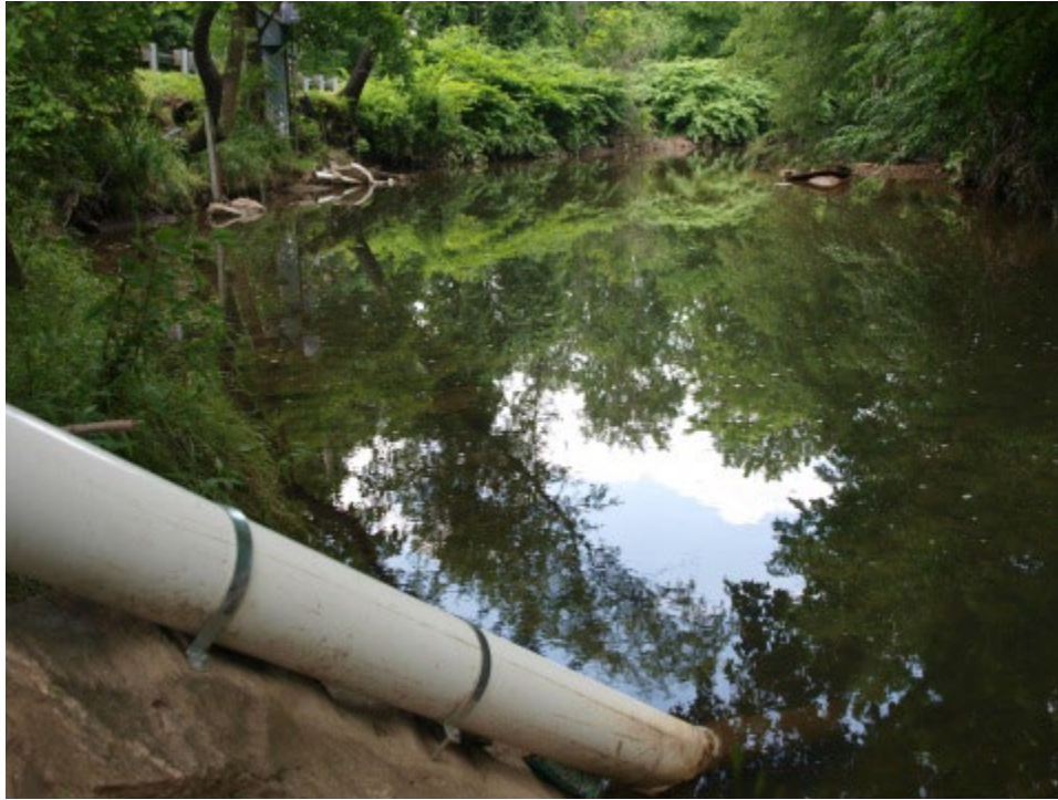
Figure 57. Gage 01465798, Poquessing Creek at Grant Ave., looking upstream
