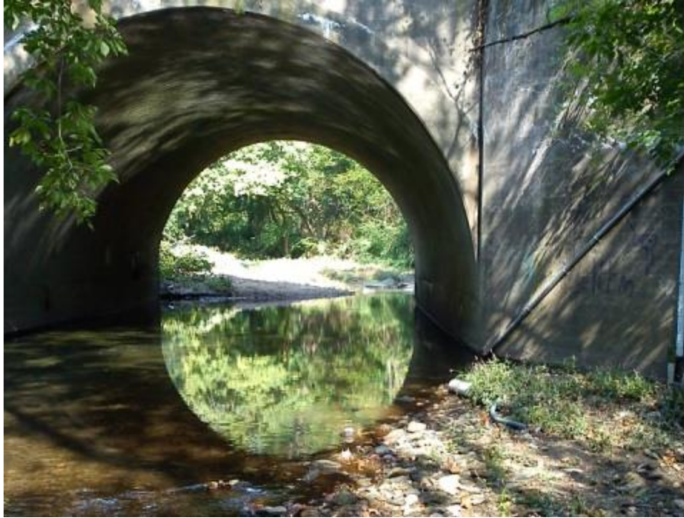
Figure 23. Gage 01475530, Cobbs Creek at Rte. 1, looking upstream
