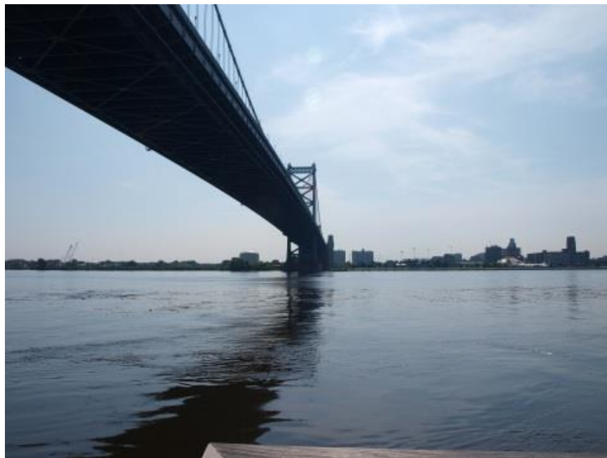
Figure 62. Delaware River at Ben Franklin Bridge, near Gage 01467200
