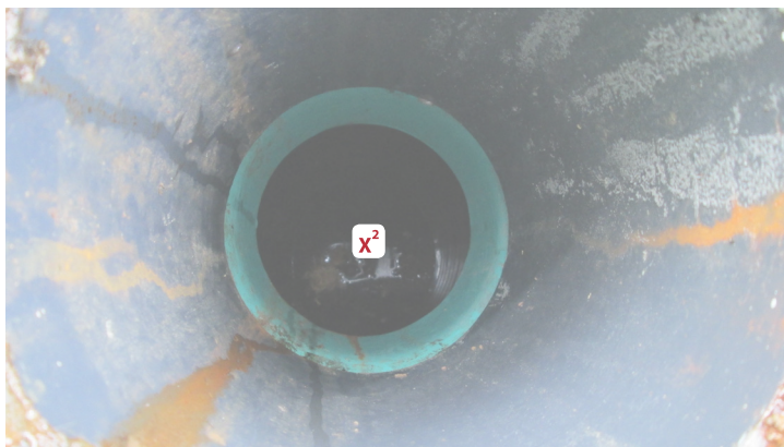
Bottom of Access Structure: bottom interior level of the structure.
