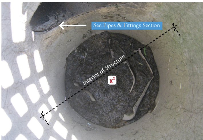
Invert of Pipe Connections and Bottom of Access Structure: bottom interior elevation of pipe, and bottom interior level of the structure.
