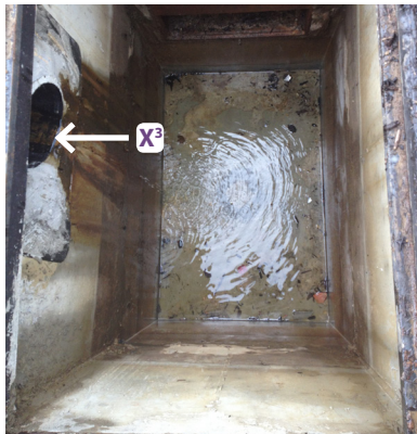
Invert: of pipe connection.
