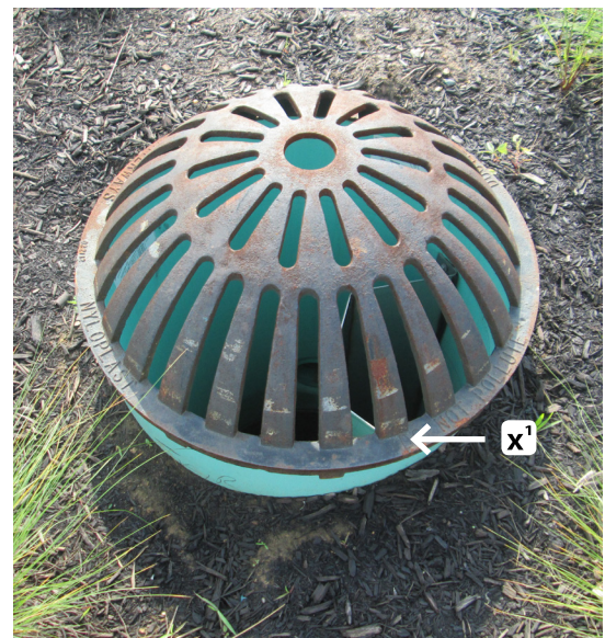
Rim elevation: the lowest level of the grate where water would enter the riser.
