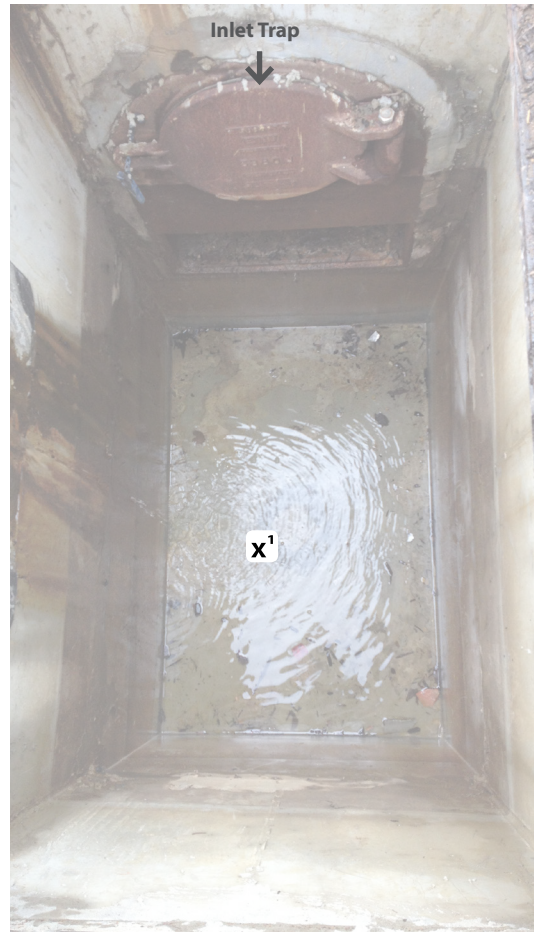
Bottom of box: Survey the bottom interior elevation of the inlet.
