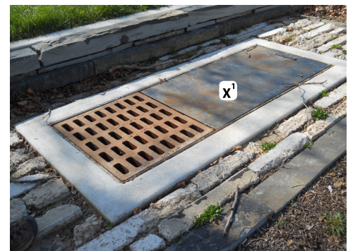
Non-Standard Inlet: dual trap inlet.
