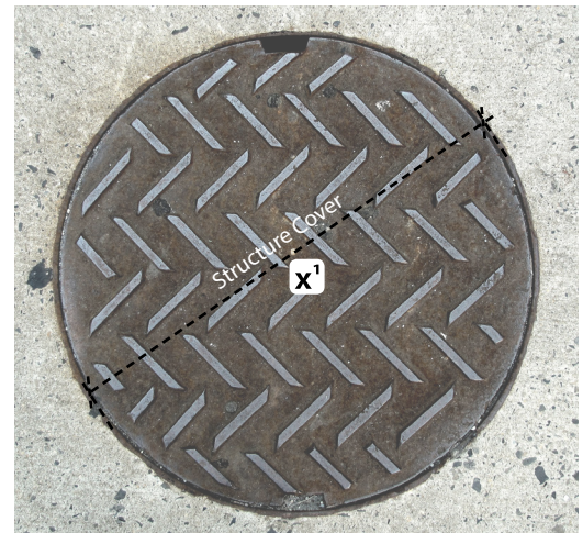
Rim Elevation: center point on top of cover or lid.
