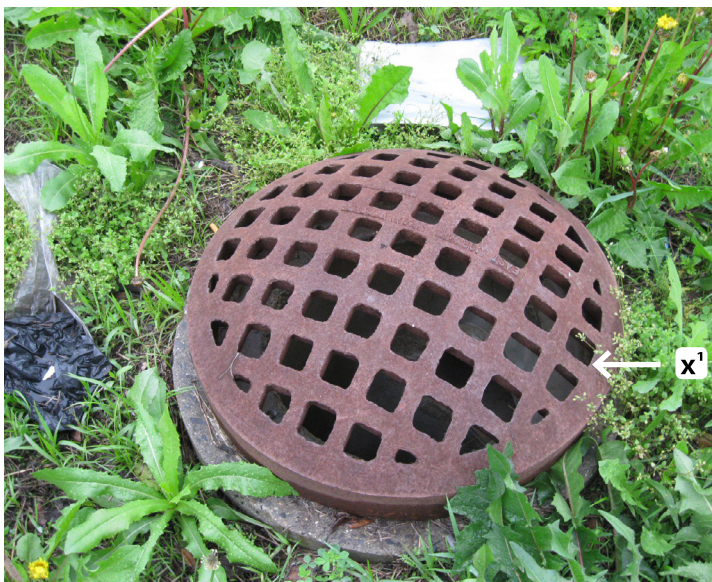
Rim elevation: the lowest level of the grate where water would enter the riser.
