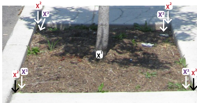
Depressed Tree Pit: location of trunk and perimeter. The tree pit will be lower than adjacent grade.
