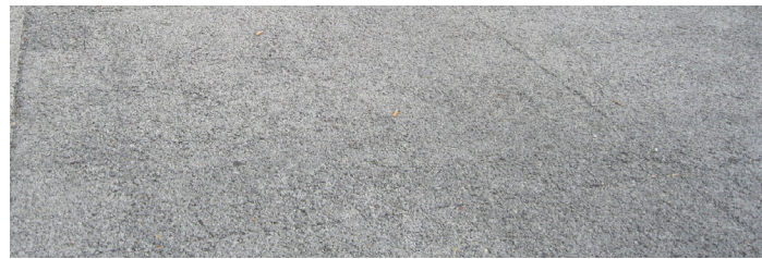
Permeable pavement surface
