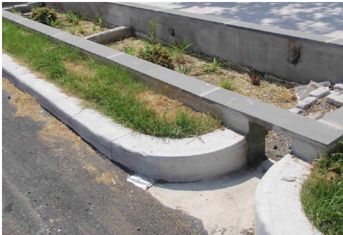
Curb Cut: along street right-of-way.
