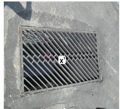
Highway Grate Inlet: survey centroid of grate.
