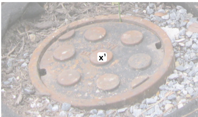
Rim of cover: center point taken on top of cover. Diameter of observation well cover to be documented.
