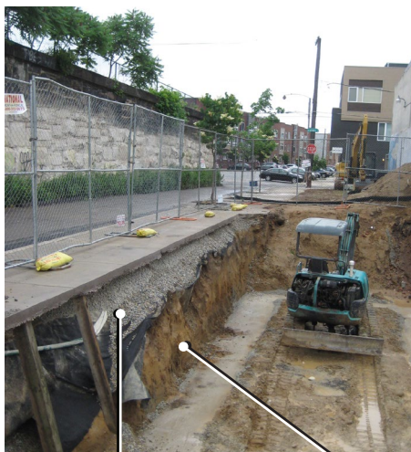
Subsurface Stone Adjacent Excavation
