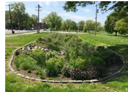
Cobble edging defines the edge of the rain garden for PWD maintenance crews and PPR mowing crews
