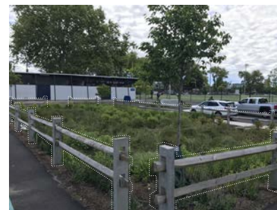
Split rail fencing deters users cutting through the system and protect against cyclists
