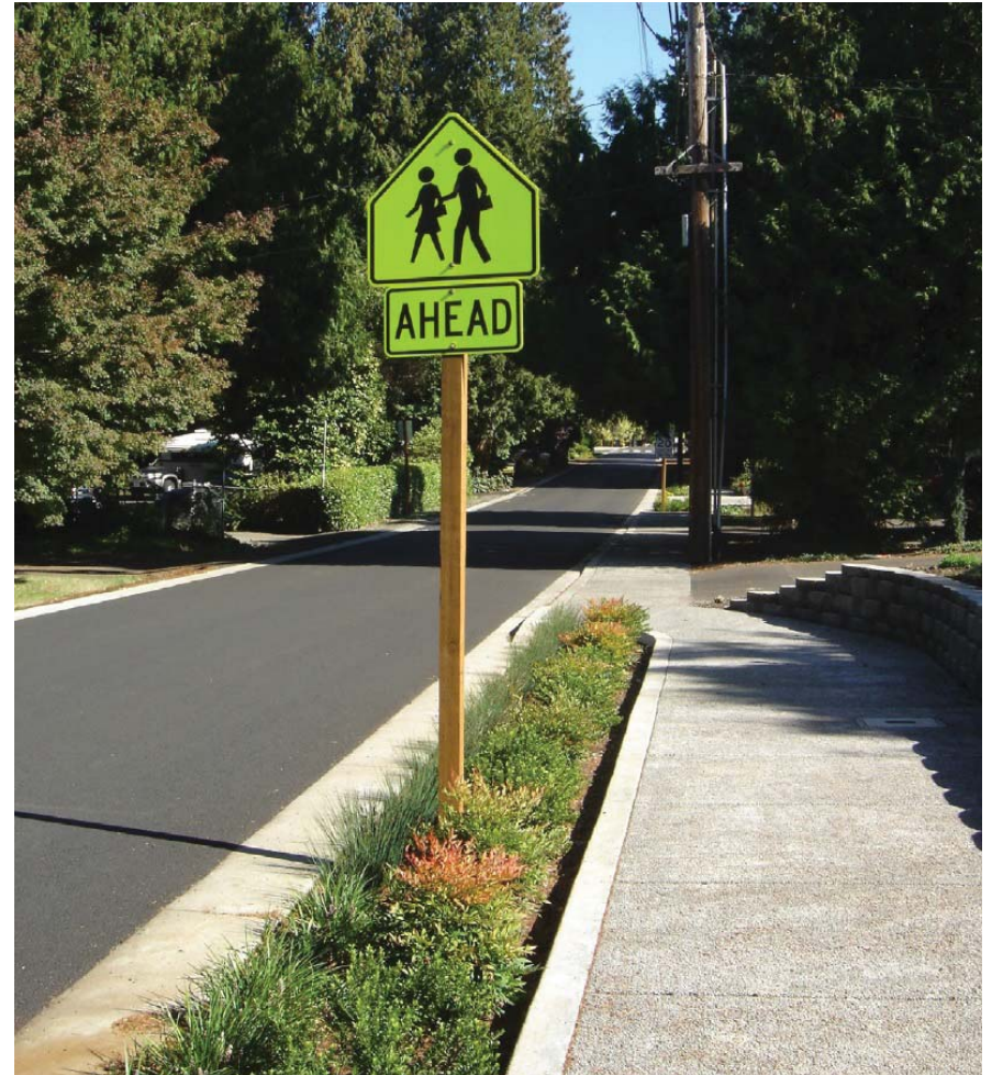
Figure 1-31. Example of a Green Gutter in Portland, Oregon (Image credit: PWD Green Streets Design Manual, 2014)
