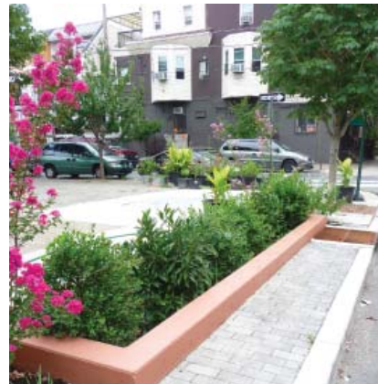
Figure 1-9. Examples of Stormwater Planters in Philadelphia
