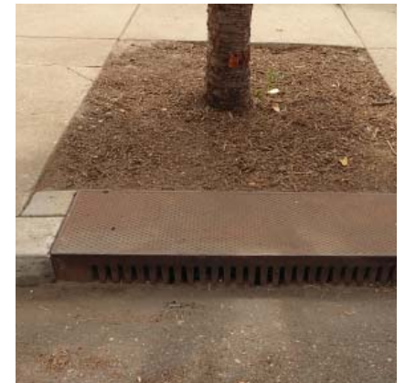
Figure 1-19. Examples of Stormwater Trees in Philadelphia
