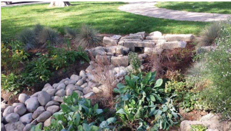
Figure 2-4. Extension of a Velocity Dissipator
