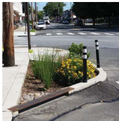
Figure 1-6. Examples of Stormwater Bump-outs in Philadelphia
