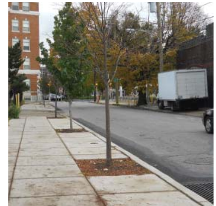
Figure 1-1. Examples of Stormwater Tree Trenches in Philadelphia
