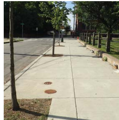
Figure 1-1. Examples of Stormwater Tree Trenches in Philadelphia
