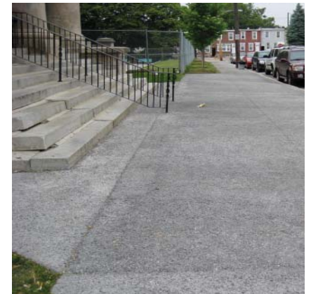
Figure 1-23. Examples of Pervious Pavement in Philadelphia
