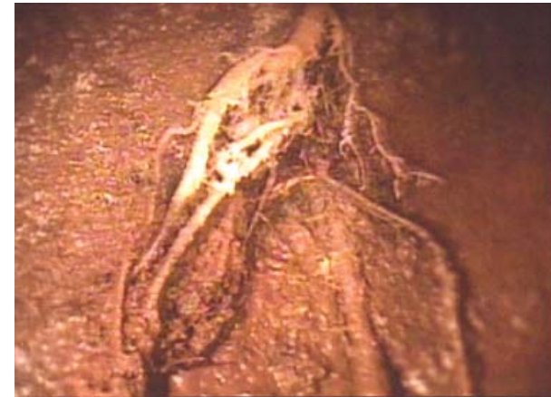
Figure 3-21. Tap Roots: Individual Roots that are Greater than \frac{1}{2} in. (10mm) Thick.
