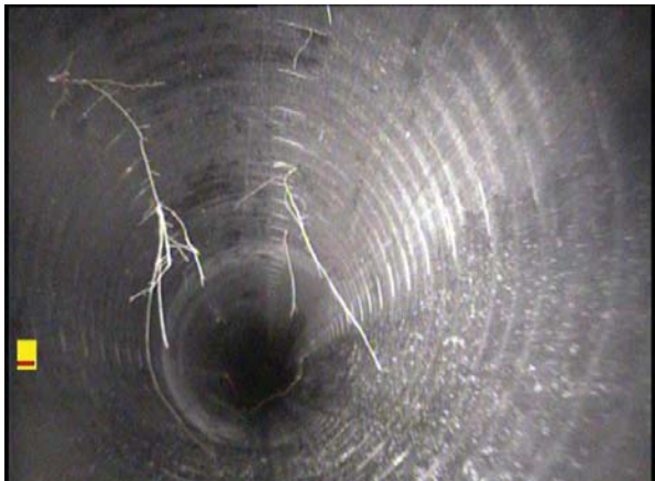
Figure 3-20. Roots - Fine: Small Diameter and Small Quantities of Roots that are Insufficient to Cause a Quantifiable Reduction of Pipe Cross-sectional Area (<5% loss).
