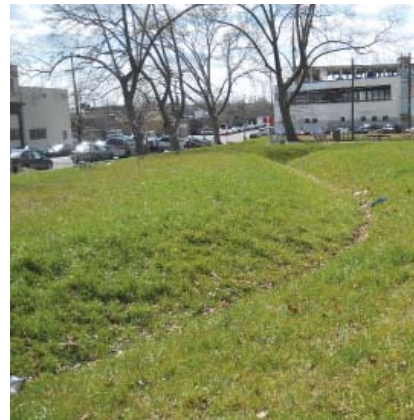
Figure 1-17. Examples of Stormwater Swales in Philadelphia
