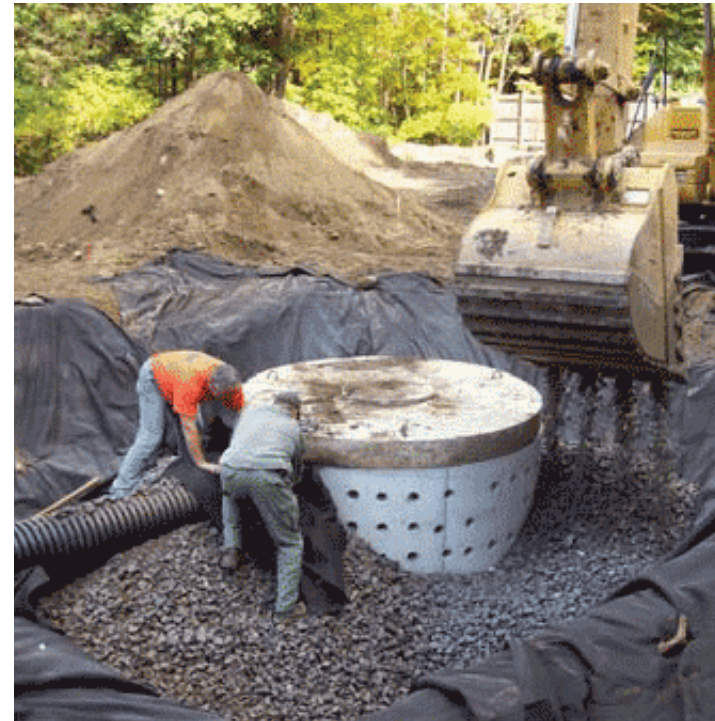
Figure 1-33. Example of a Drainage Well Installation (Image Credit: Lake George Association)
