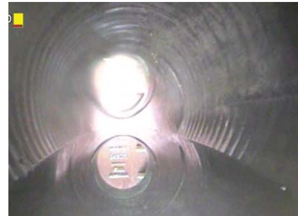
Figure 3-25. Water Level: the Depth of Water at the Observed Point in the Pipe (Includes Flowing and Stagnant Water). Water Level Sag Occurs when the Grade of the Pipe is Poor.
