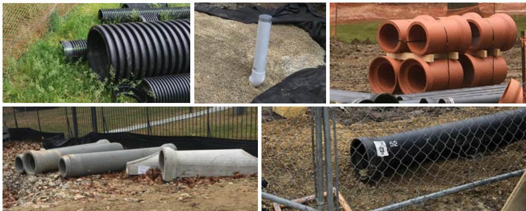
Figure 46: Images showing the various types of piping used in PWD's GSI systems. From top left to bottom right: HDPE, PVC, VCP, RCP, ductile iron.
