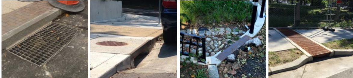
Figure 45: Images showing the various types of inlets to convey runoff to GSI systems. From left to right: a green highway grate inlet, a green city inlet, a curb cut with wheel guard and energy dissipator, and a trench drain.
