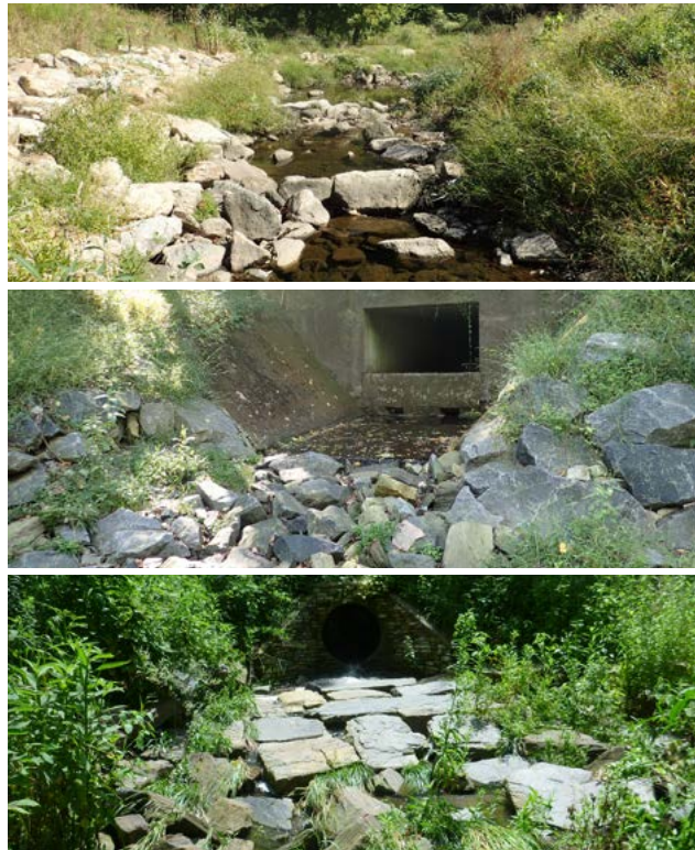
Figure 37: Images showing types of energy dissipation at stream outfalls.
