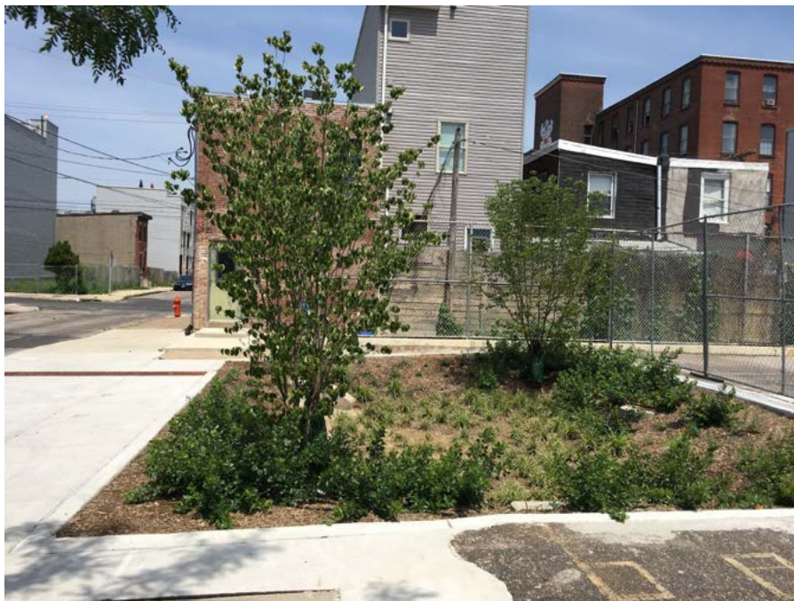
Figure 30: Example of flat grade adjacent to sidewalk to protect SMP from erosion.
