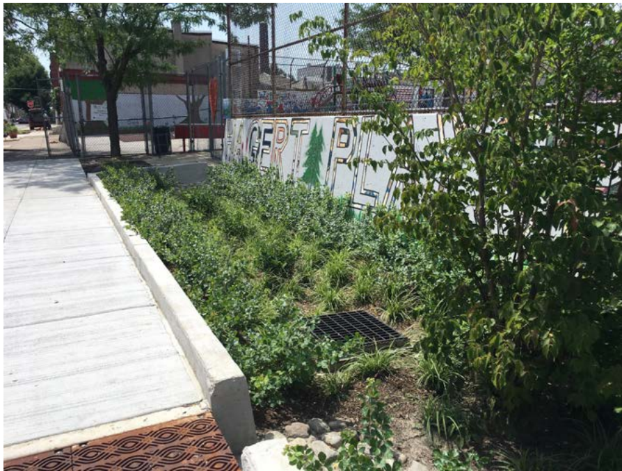
Figure 29: Example of curbing to protect SMP from erosion.
