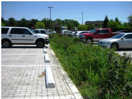
SOUTHWEST TREATMENT PLANT RAIN GARDEN
