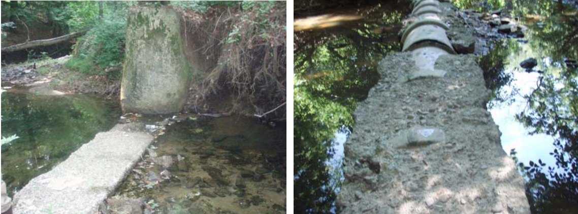
Figure 2-11: Example of a pipe assessed in infrastructure trackdown.
