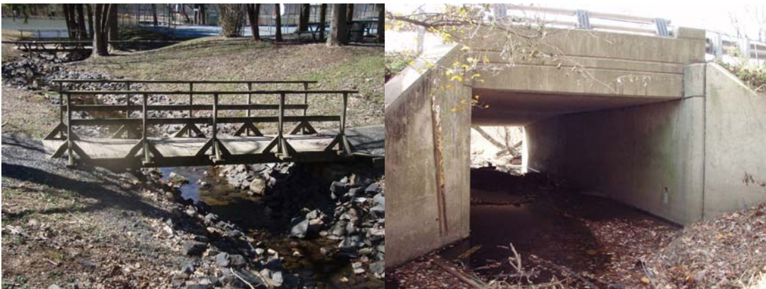
Figure 2-6: Examples of bridges assessed in infrastructure trackdown
