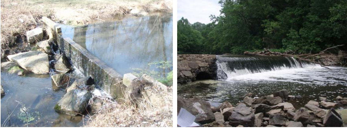
Figure 2-9: Examples of dams assessed in infrastructure trackdown.
