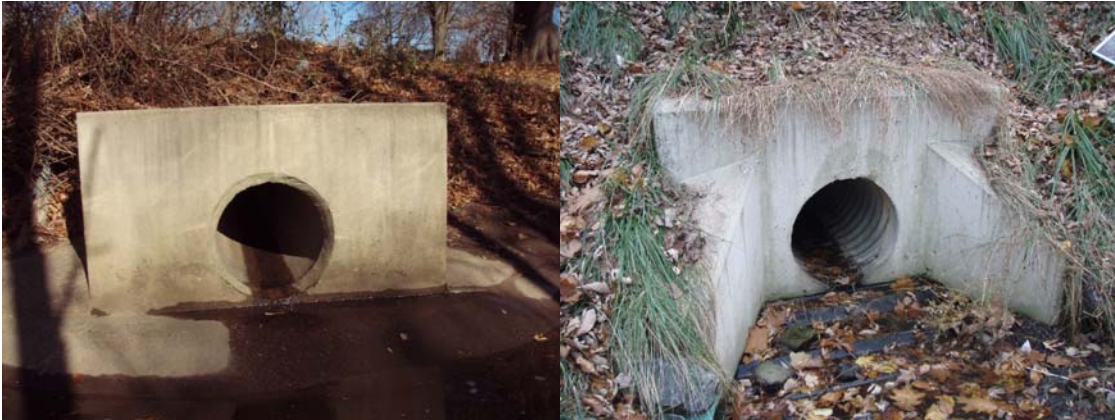
Figure 2-5: Example of an outfall point assessed in infrastructure trackdown
