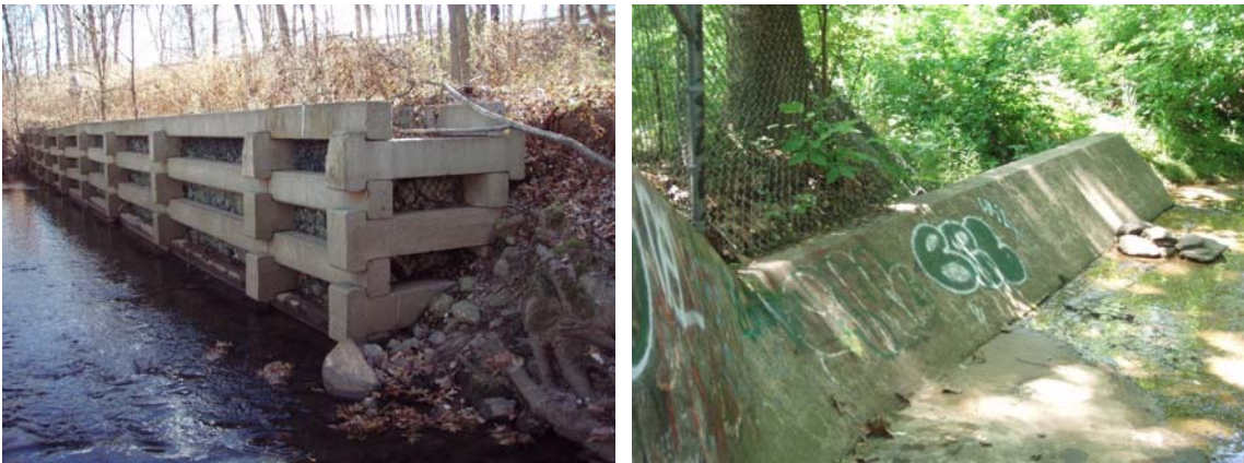
Figure 2-10: Examples of channels assessed in infrastructure trackdown.
