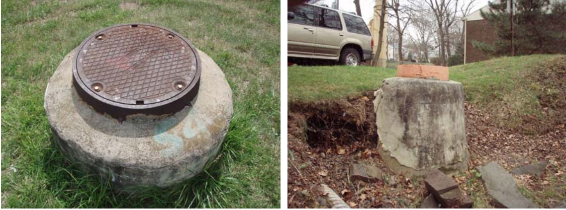
Figure 2-7: Examples of manholes assessed in infrastructure trackdown.
