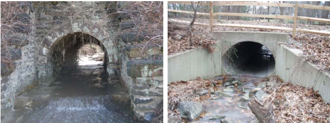
Figure 2-8: Examples of culverts assessed in infrastructure trackdown.
