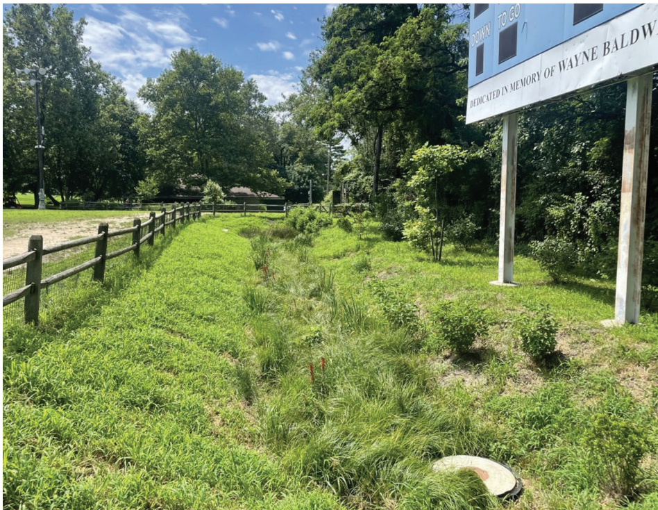
This large rain garden manages stormwater runoff from the sports field (July, 2023)
