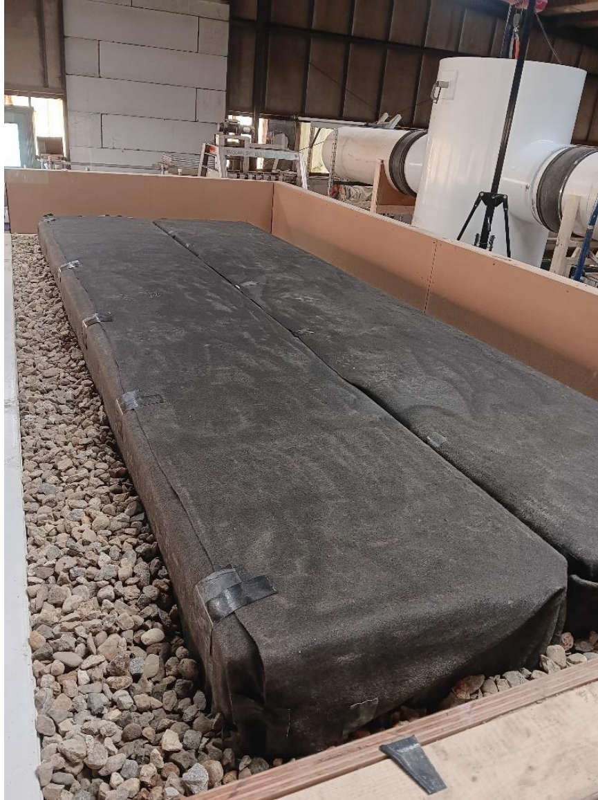
Figure 8 StormBrixx Installation
