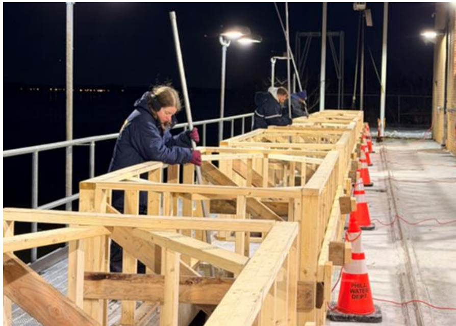
Breaking down ice to keep drinking water flowing – icy conditions make it harder to intake water from the rivers for treatment
