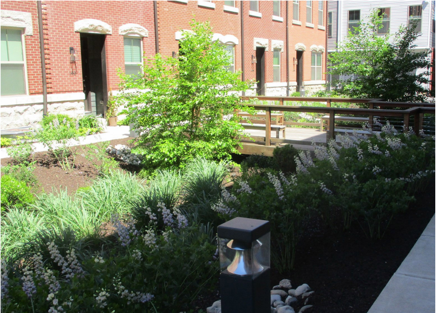
An example of a typical bioretention basin in Philadelphia
