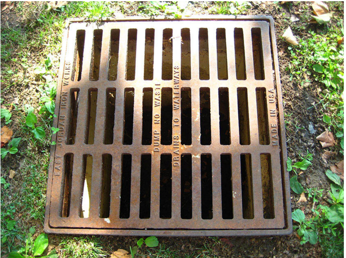
An example of an inlet in Philadelphia
