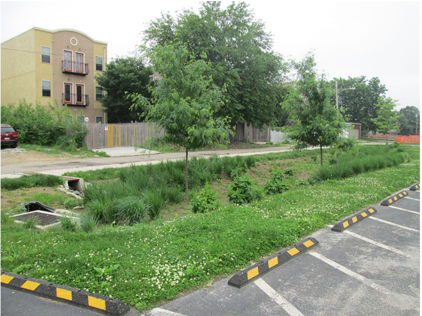
An example of curbless parking lot design in Philadelphia
