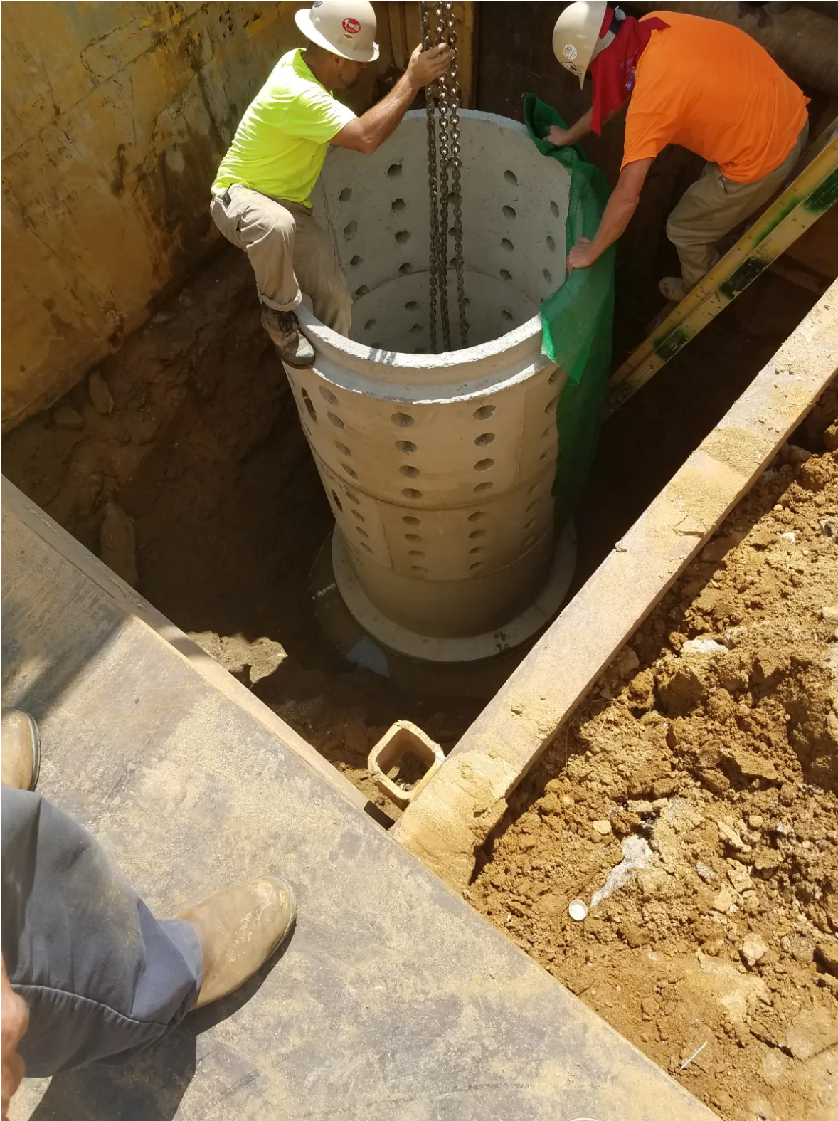
An example of a drainage well installation in Philadelphia
