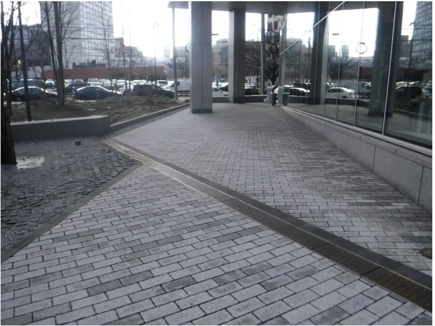
An example of permeable pavers in Philadelphia
