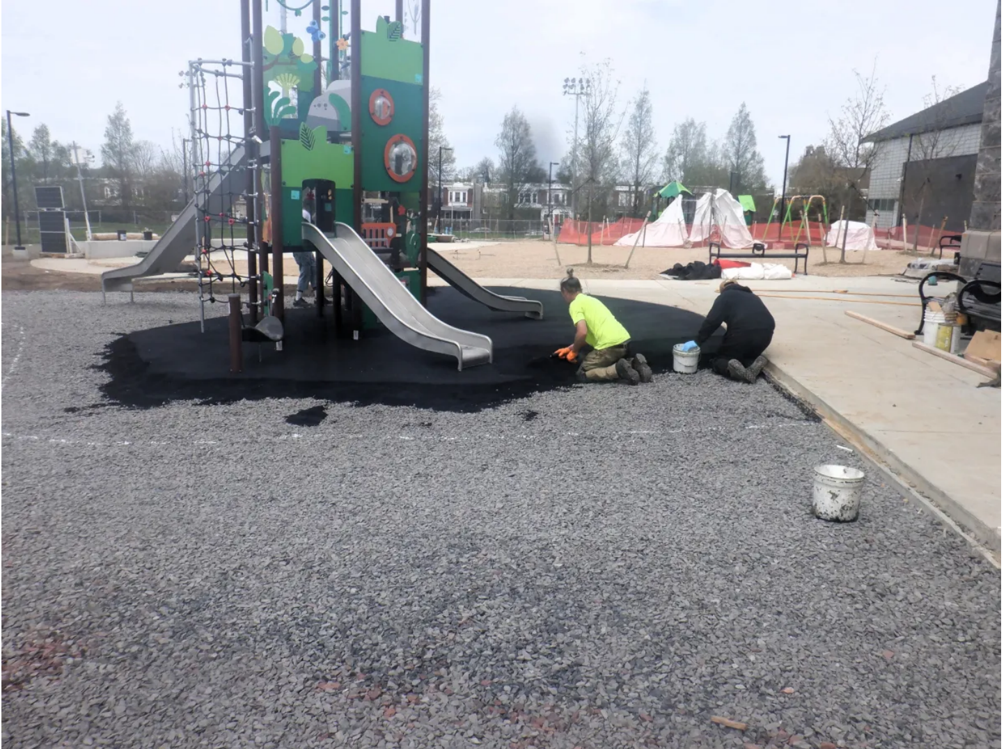
An example of a porous safety surface installation in Philadelphia
