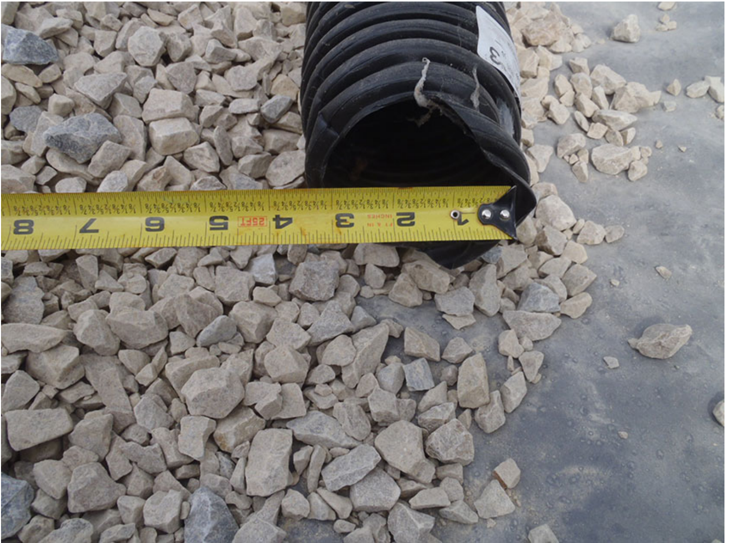
An example of pipe diameter measurement during construction in Philadelphia
