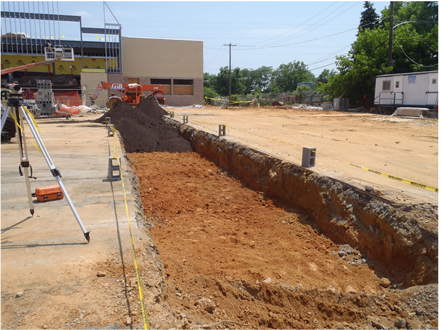
An example of SMP installation in Philadelphia
