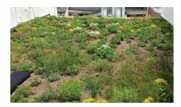
**Green Roofs:** A green roof is a roof that has been covered with vegetation to provide stormwater management.
