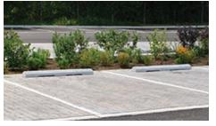
**Permeable Pavement:** A pavement system that allows water to infiltrate into the ground. Shown here as parking spaces.
