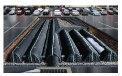
**Subsurface Storage:** Underground basins that collect runoff underneath a paved surface.
