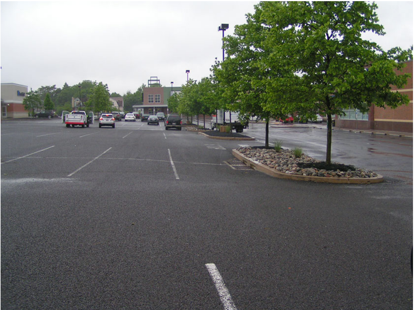
The Philadelphia Water Department includes certain types of porous pavement systems as DIC.
