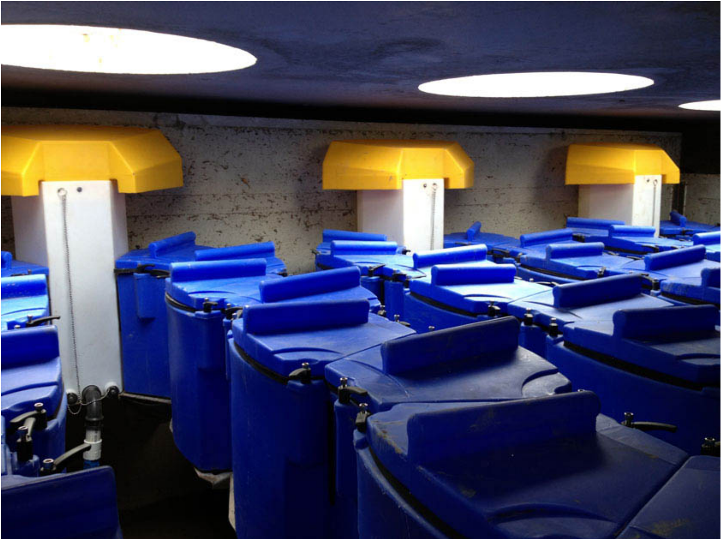
An example of a media filter in Philadelphia
