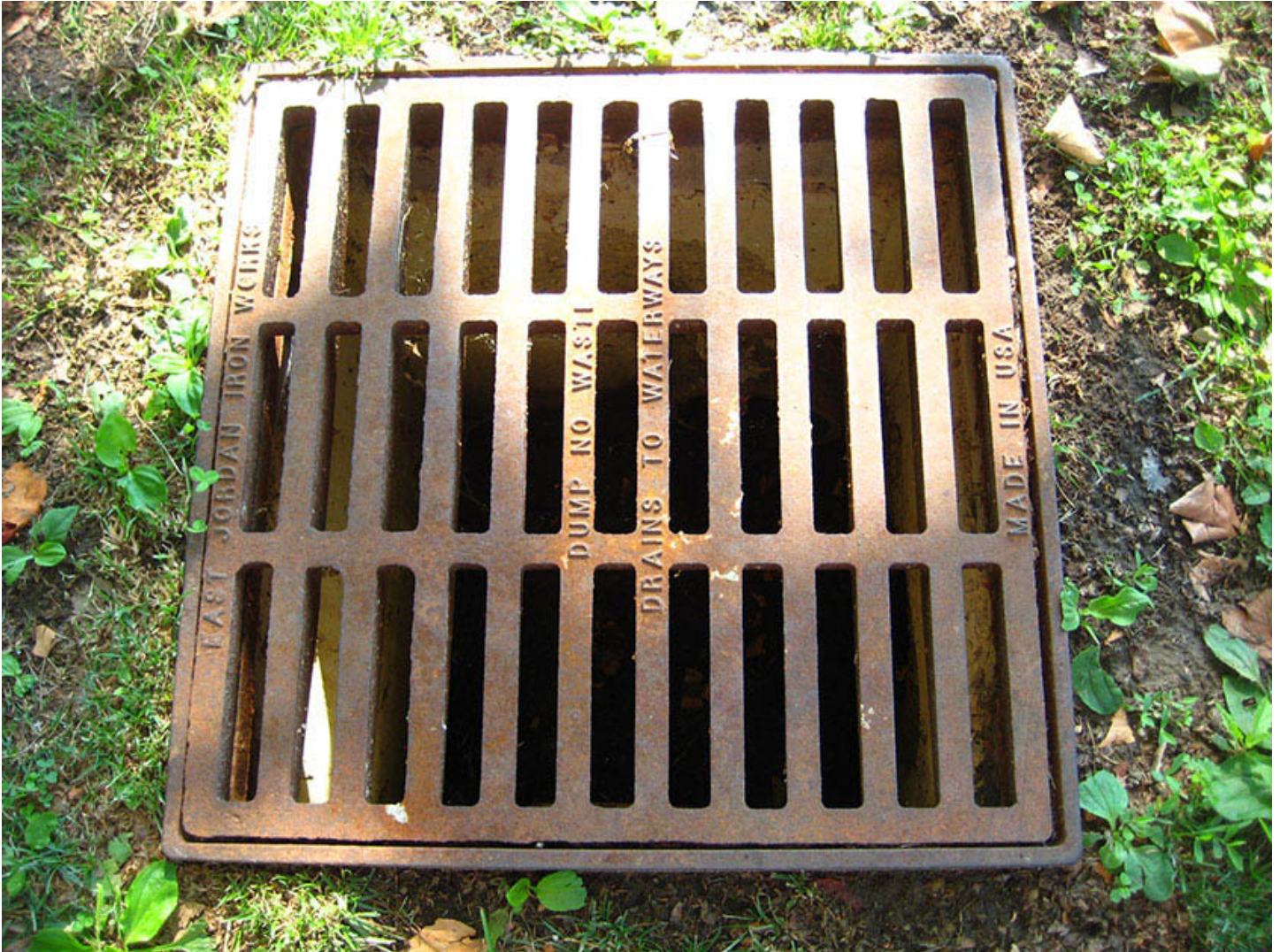
An example of an inlet in Philadelphia
