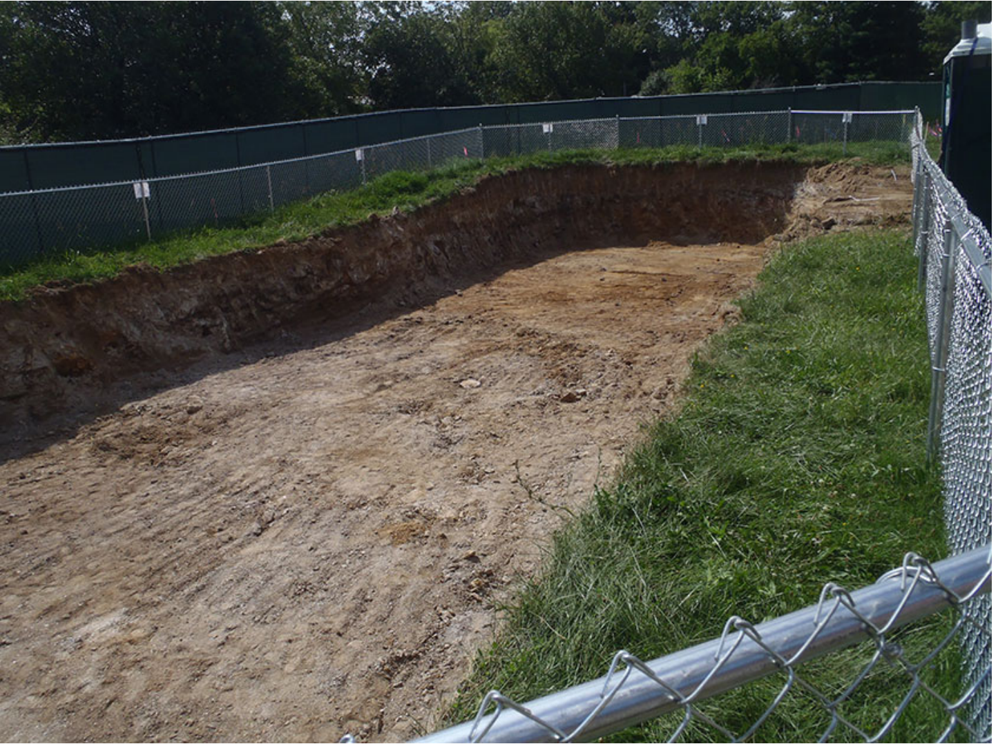
An example of infiltration area protection during construction in Philadelphia
