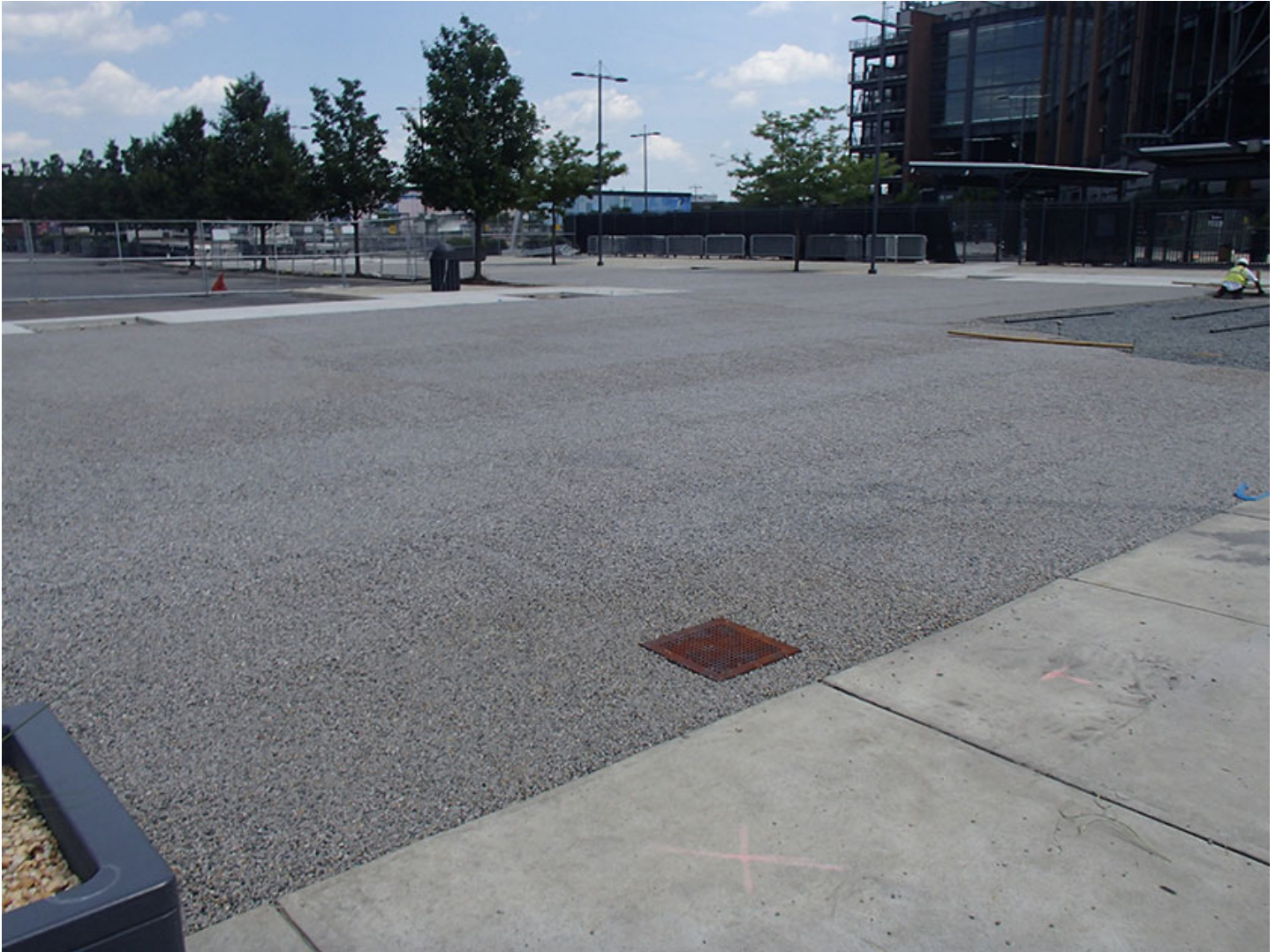
An example of a porous asphalt installation in Philadelphia
