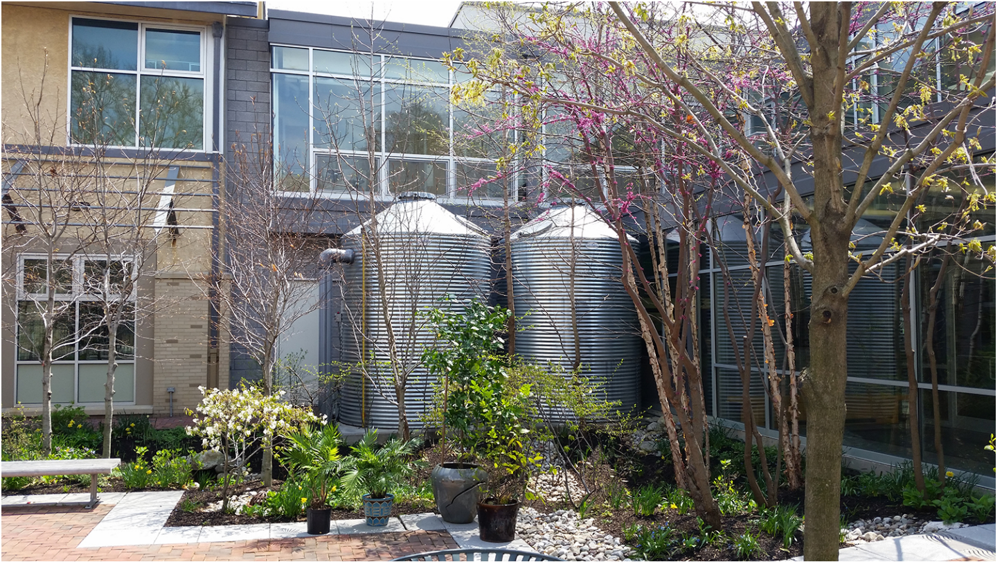
An example of a surface cistern in Philadelphia
