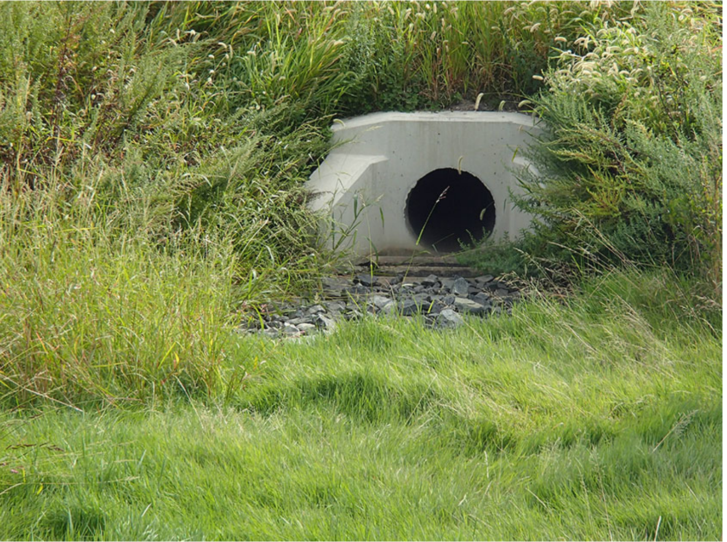
An example of a riprap apron in Philadelphia
