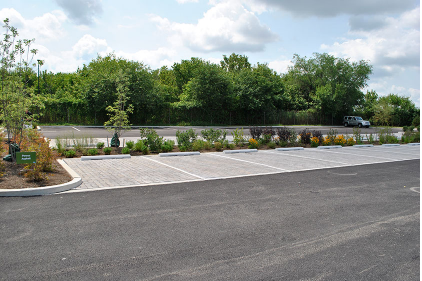
An example of porous paver parking spaces in Philadelphia
