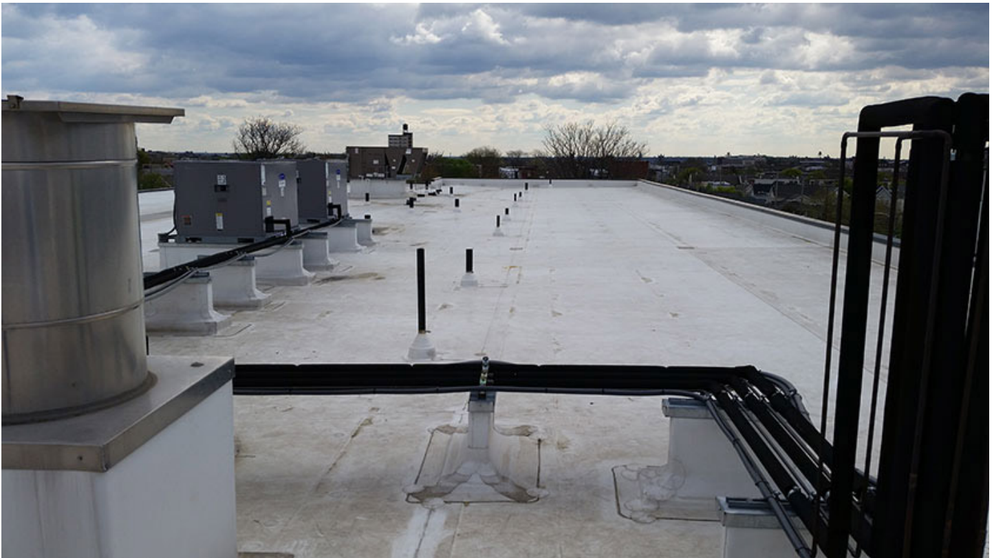
An example of a blue roof in Philadelphia
