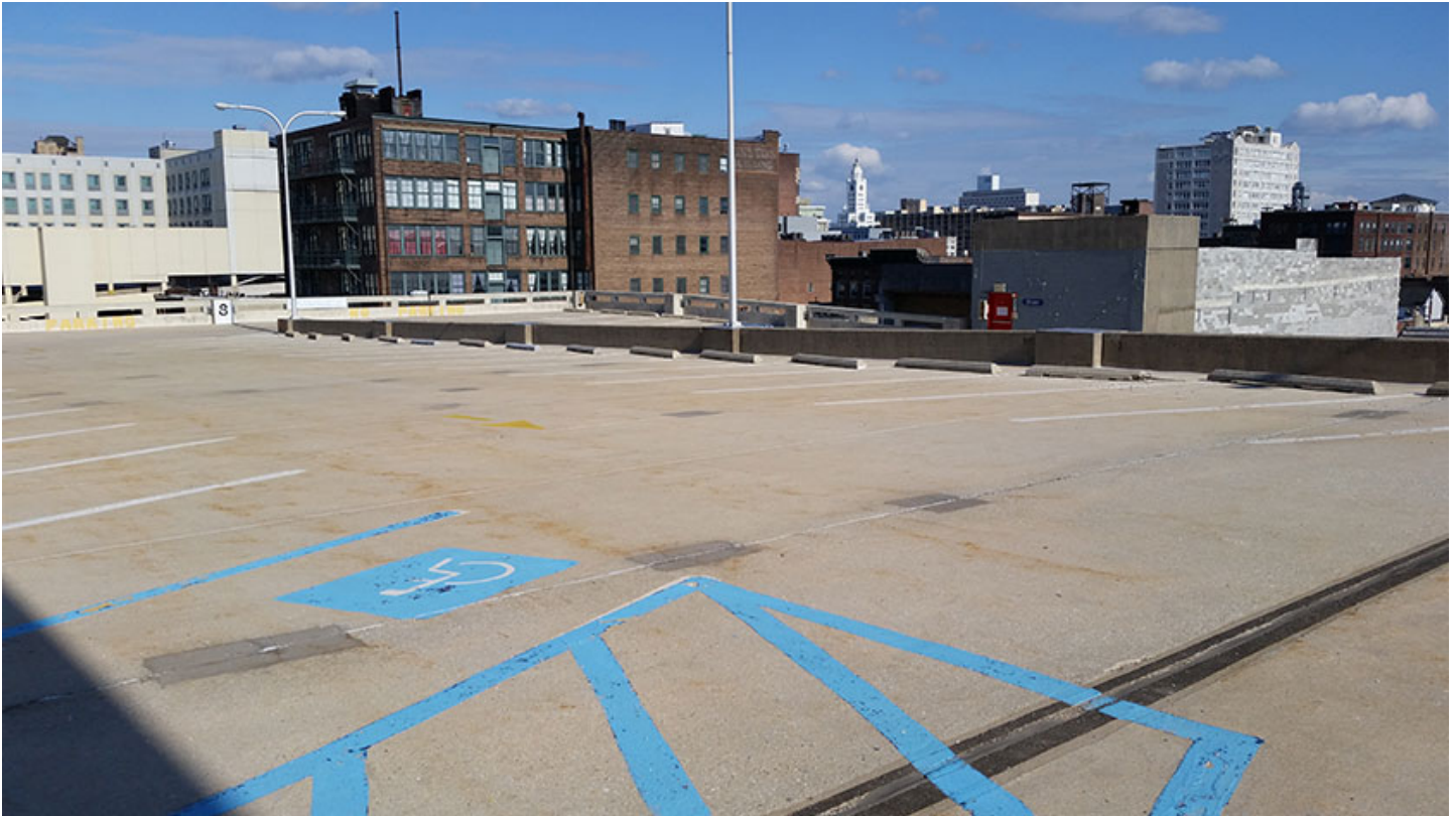
This Philadelphia parking garage with rooftop vehicular access does not qualify for roof runoff isolation.
