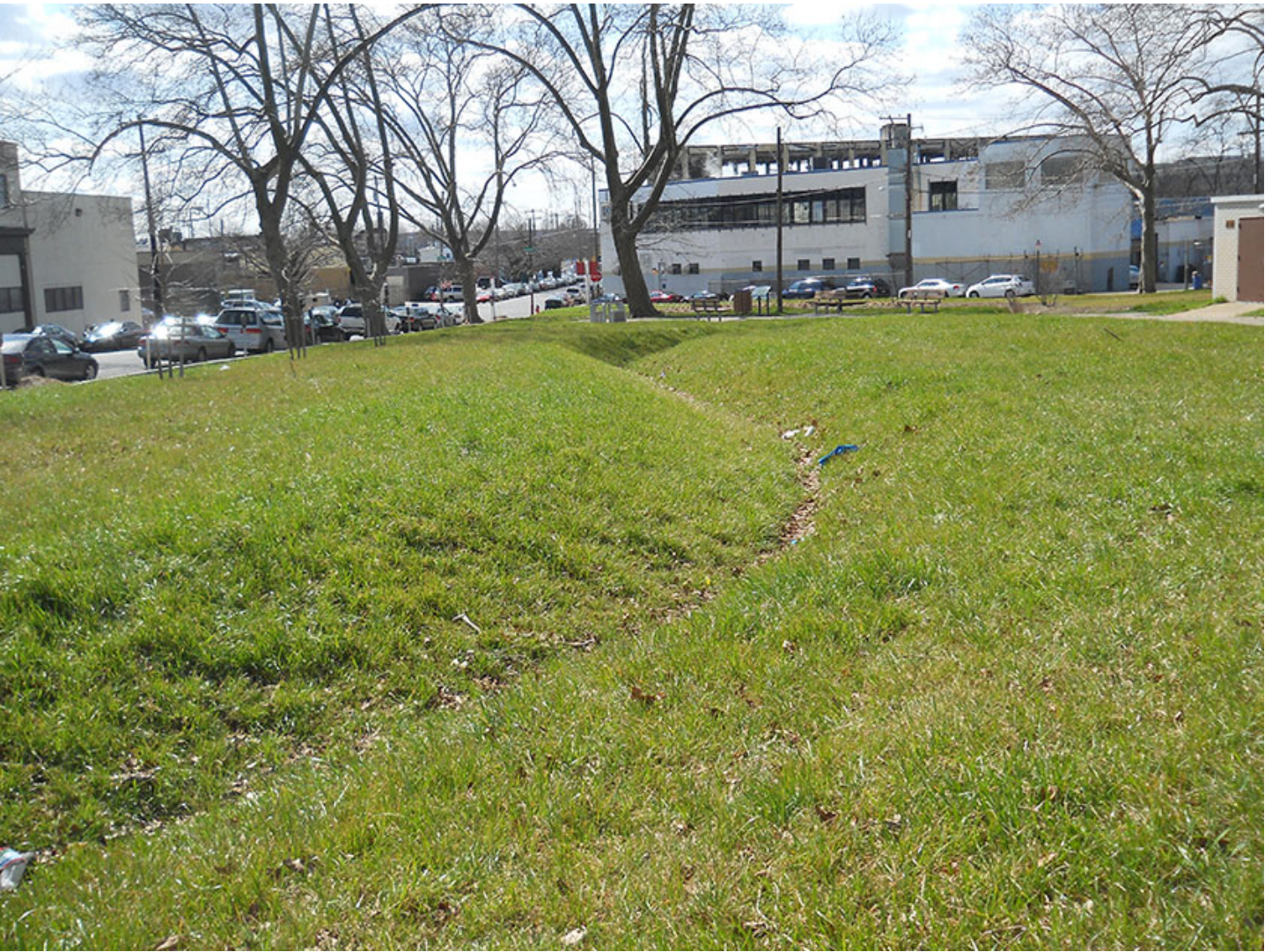
An example of a swale in Philadelphia
