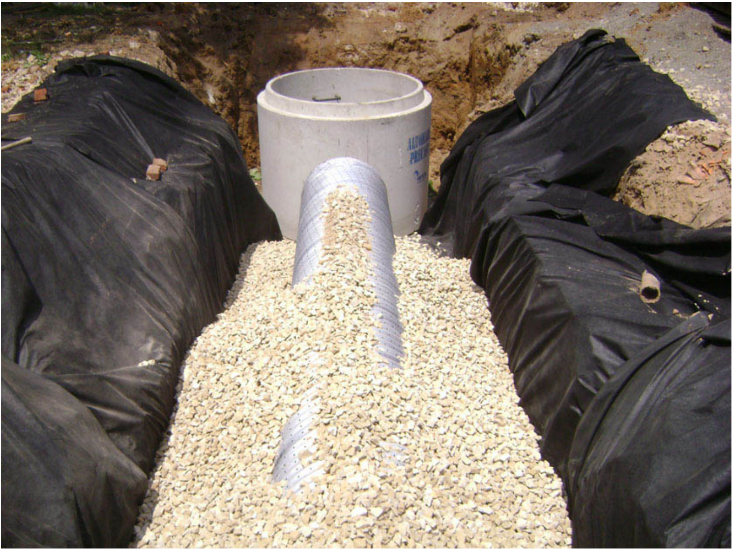
An example of an outlet control structure installation in Philadelphia
