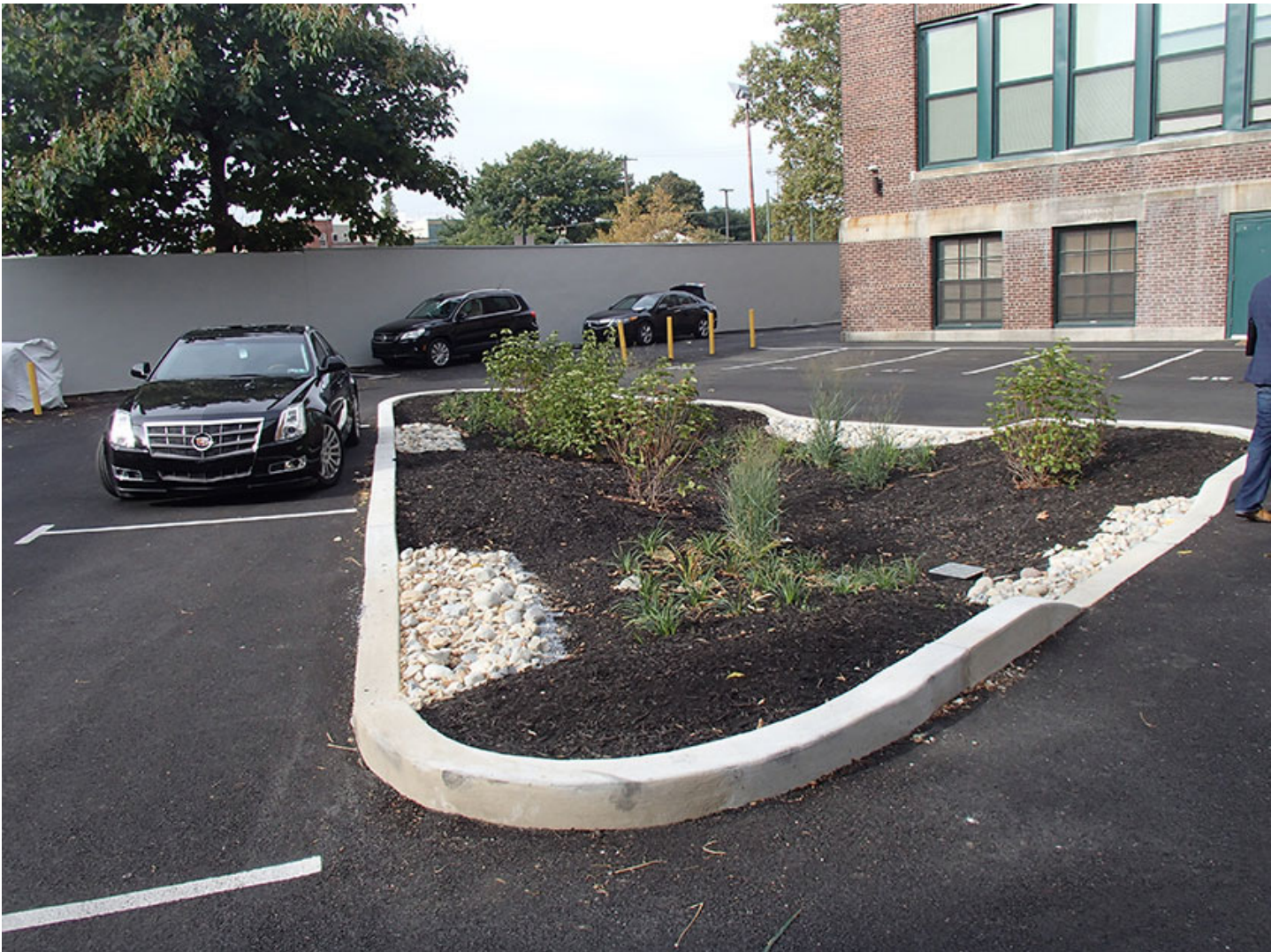
An example of filter strips in Philadelphia
