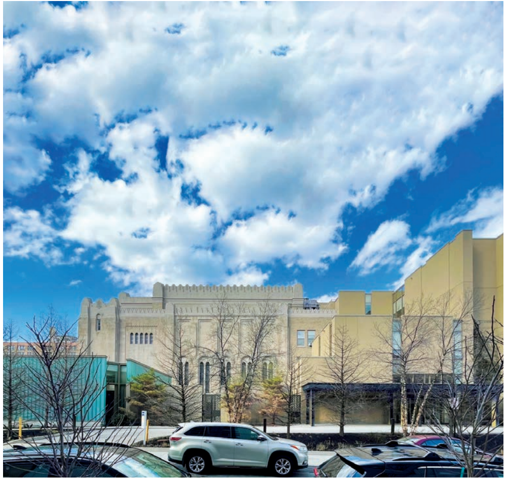
At Congregation Rodeph Shalom, located on North Broad Street between Green and Mt. Vernon Streets, new landscaping and repaved surfaces cover a large subsurface basin managing stormwater. Photo © Philadelphia Water Department
