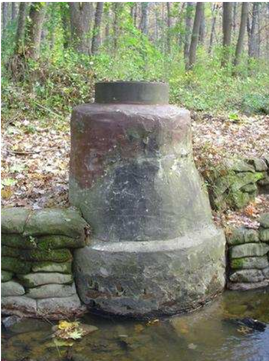
Figure 8 - Example of a manhole collected during infrastructure assessment
