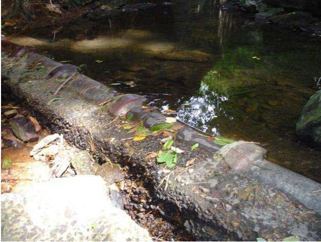
Figure 13 - Example of a pipe collected during infrastructure assessment
