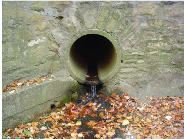
Figure 6 - Example of an outfall collected during infrastructure assessment
