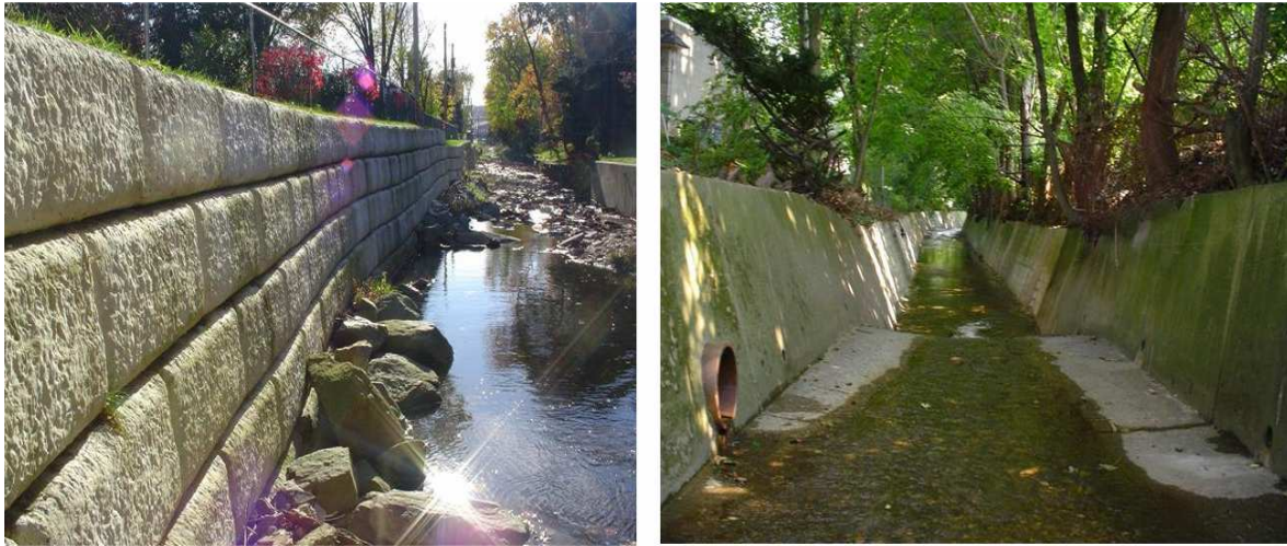
Figure 11 - Examples of channels collected during infrastructure assessment
