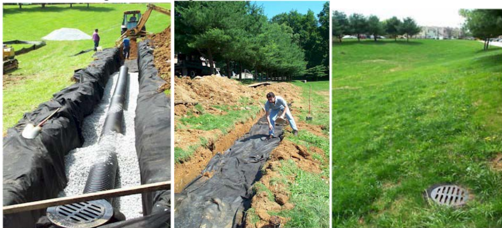
Figure 3: Example of Infiltration Trench Installation
